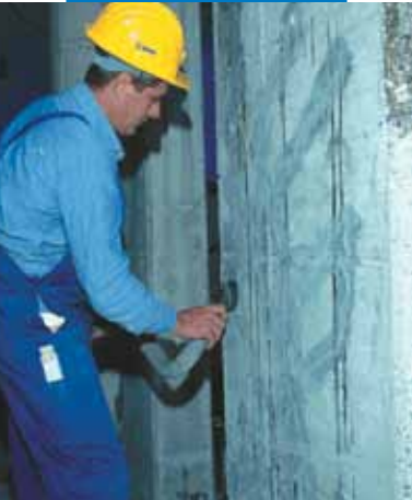
Preparing the substrate
