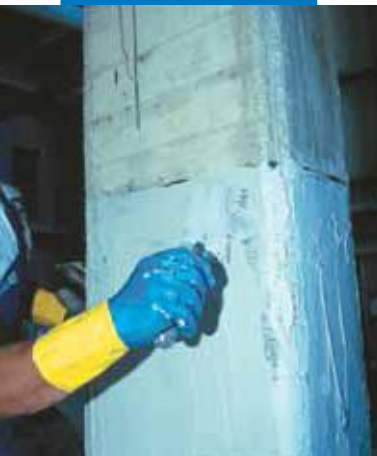
Levelling with MapeWrap 11 or MapeWrap 12
