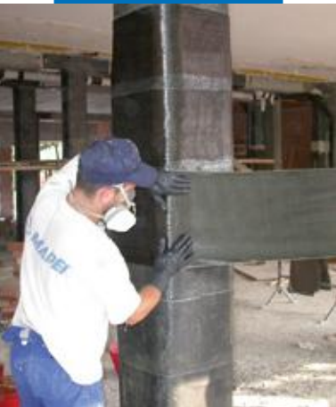
Confinement of a column with MapeWrap C UNI-AX HM
