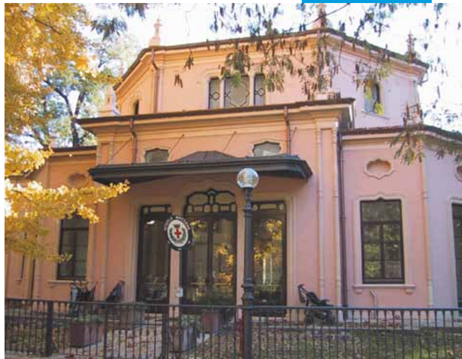
An example of an application of Silexcolor Tonachino . Nursery School - Porta Venezia Gardens (Milan) - Italy
