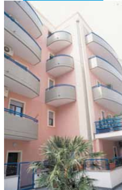
An example of an application of Silexcolor Tonachino - Rosa Residence Apartments - Gallipoli (Lecce) - Italy
