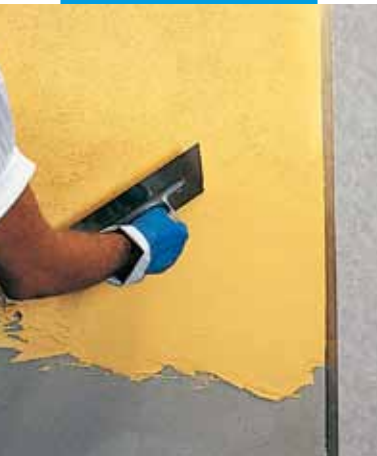
Applying Silexcolor Tonachino with a trowel
