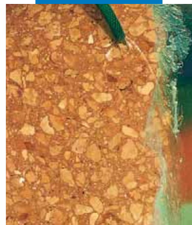
Applying WallGard Graffiti Remover Gel on natural stone
