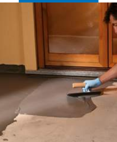
Waterproofing of terraces by trowel
