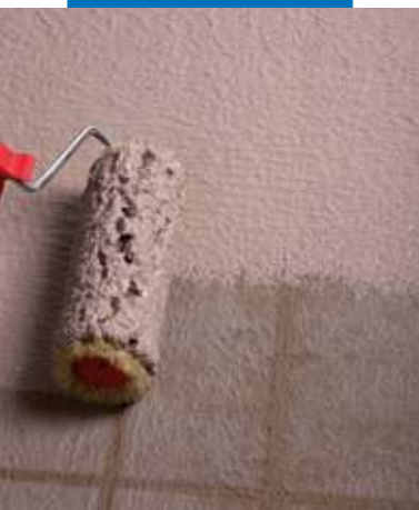
Waterproofing of details by roller
