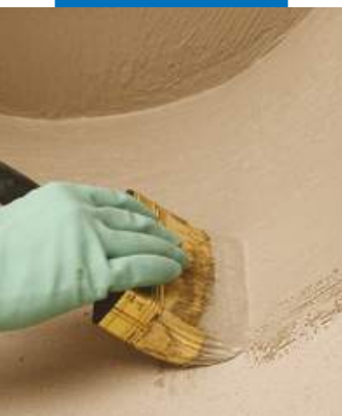
Waterproofing of details by brush
